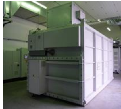
DFC®400 EU MCFC-Fuel Cell Power Plant 400 kW; 400 V; 50 Hz
